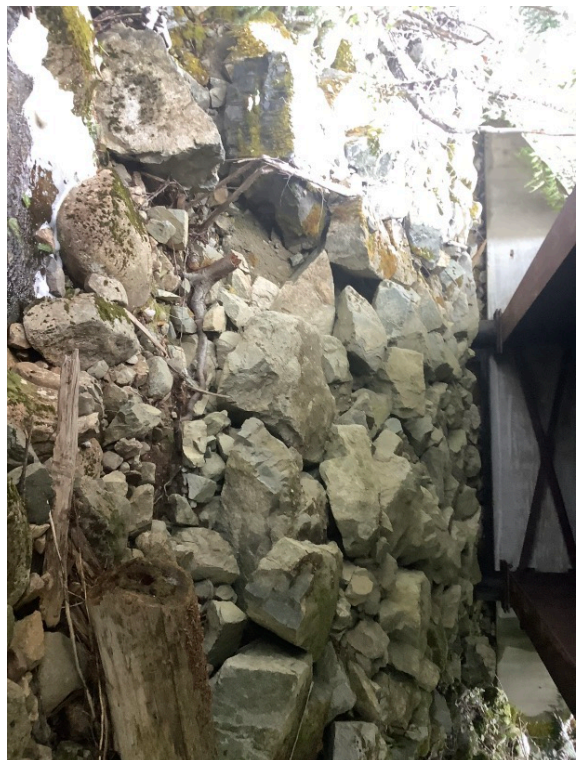
Right Bank Abutment when facing downstream
